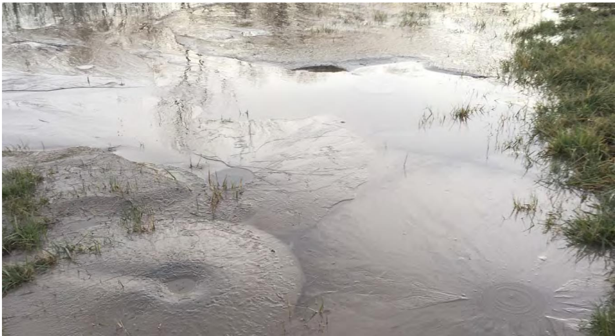
Figure 8 - Sand boils approximately 1,200 feet landward of the levee with water still seeping through near Cairo, IL (Rutherford et al., 2016)
