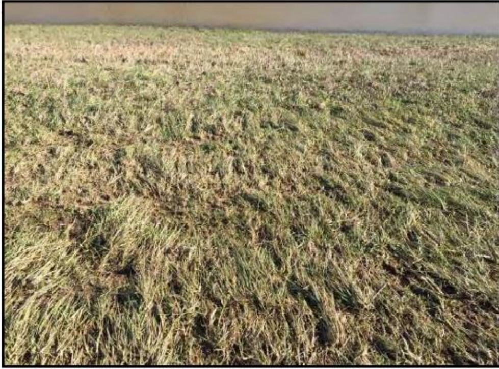
Figure 4 - vegetative cover laid down and acting as an armor on the landside slope of the levee near Olive Branch, IL (Rutherford et al., 2016)
