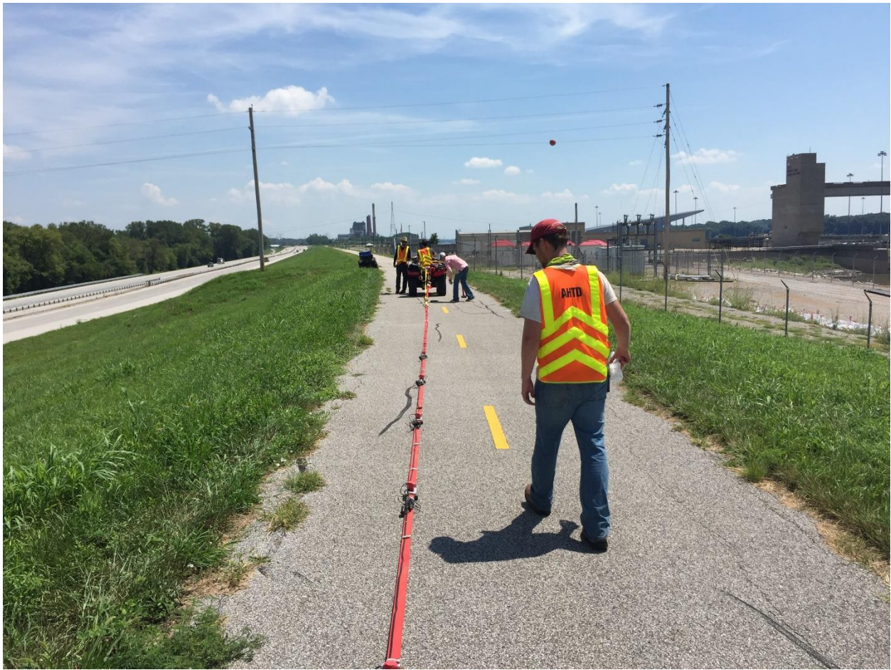
Figure 13 - Use of land streamer to collect seismic wave velocity data on top of a levee in Mel Price lock and Dam in Edwardsville, IL
